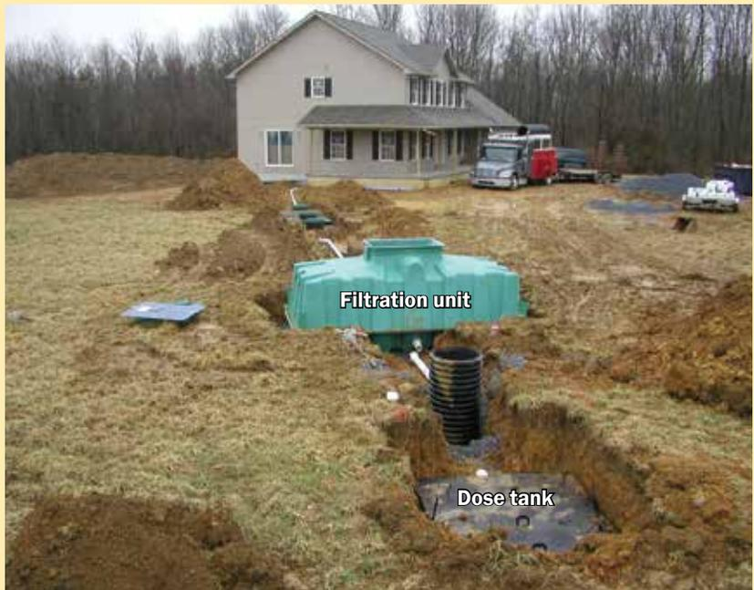
**Conventional onlot sewage system components may include, clockwise from top left, a two-series septic tank, a trench absorption field, or a filtration unit and dose tank. (Photos courtesy of DEP.)**
