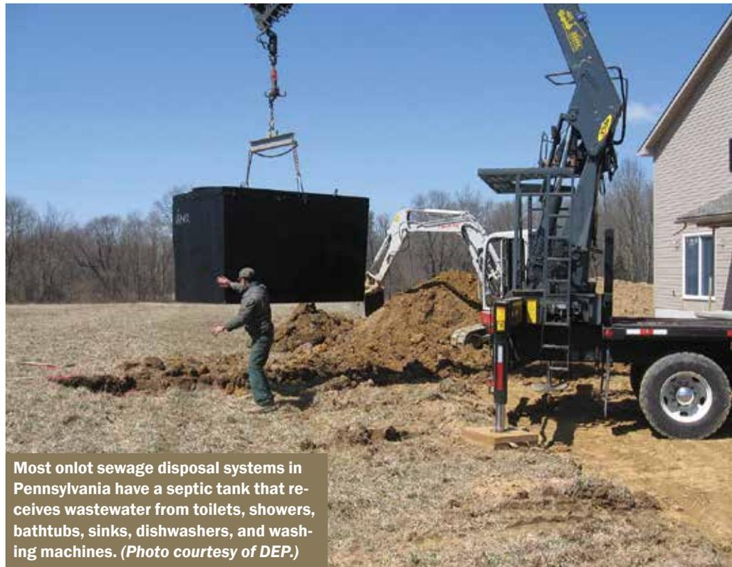
Most onlot sewage disposal systems in Pennsylvania have a septic tank that receives wastewater from toilets, showers, bathtubs, sinks, dishwashers, and washing machines. (Photo courtesy of DEP.)
